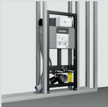
Dry-wall installation in a plasterboard wall frame
